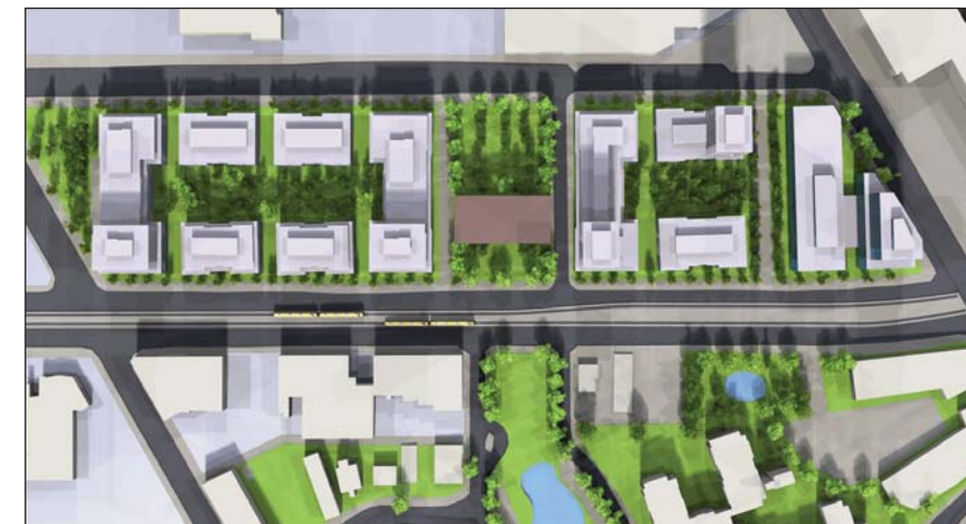
An aerial rendering of the redeveloped large front and back site close to Fairview. The size of the block is large enough that development could address both the front and rear of the block.
